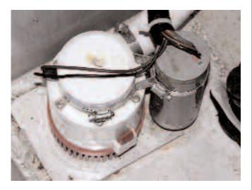
A high-capacity bilge pump mated with a durable, reliable reed float switch installed in the bilge of an aluminum trawler. The wiring is well secured and chafe protected, and the pump rests on a small platform, reducing the likelihood of debris fouling.
