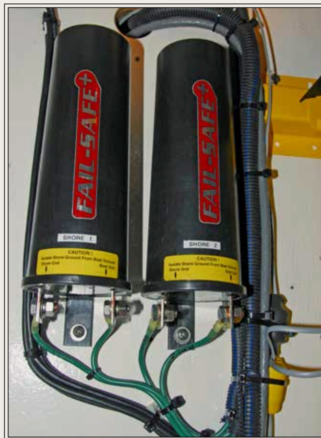
Galvanic isolators are used to protect boats that are berthed in proximity of each other from damage when they're plugged into shore power (above, left). An aluminum bracket is being eaten away as water drips on it from a bronze pump (top, right). A metal shaft log corroded because the alloy it was made of contained too much zinc.
