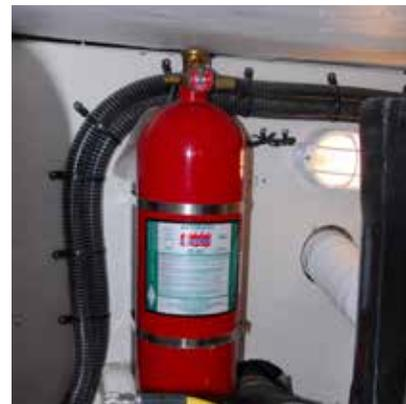
*A fire extinguishing system must be capable of flooding the space it protects. Combining two smaller bottles (top) would not comply with standards unless each could flood the space. Tanks should be mounted as high as possible in the engine room and away from ventilation systems (above, left). Installing the bottle's heat-sensitive nozzle close to the overhead ensures it will trigger quickly in case of a fire.*
