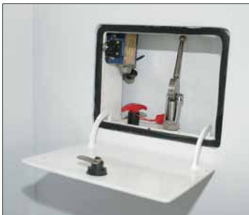
Left —Whenever possible, manual discharge handles should be installed in plain view. If one is placed in a locker, clearly label it to indicate its presence. Center —The exposed manual discharge handle is missing its arming pin. Right —Be certain you and your customer understand that the indicator light goes out once the system has discharged.
