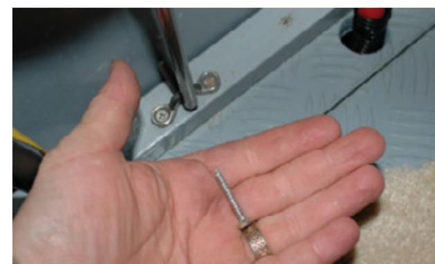
Top: While web straps can be used to secure batteries, they must be durable, robust and properly secured to the shelf or vessel. Fasteners passed directly through a strap are inappropriate for the loads that are involved. Above: Ideally, hardware used for battery security should be through-bolts rather than tapping screws. Where tapping screws are used, they must be large enough to support the load and the substrate into which they are screwed must be capable of retaining them without failure.
