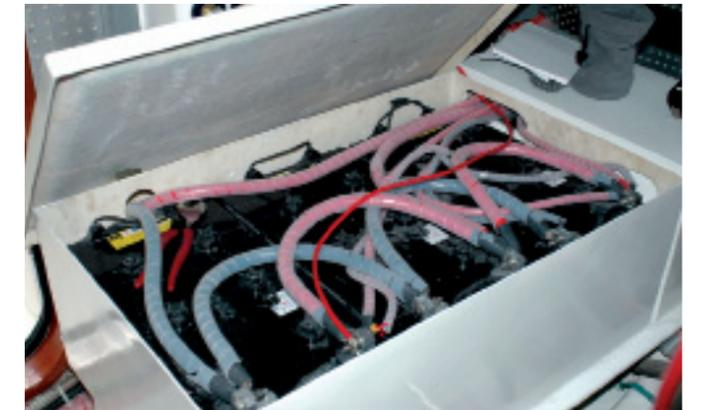
Left: While this large battery bank is easily accessible for routine inspections, it does contain a flaw; inverters should not be installed directly over batteries. Right: Batteries require ventilation for two purposes: to release hydrogen gas and to dissipate heat. This installation is conducive to neither. The "shoebox" lid will trap hydrogen gas while tightly packed batteries make heat dissipation problematic. Additionally, the tool left atop the battery presents a short circuit risk.
