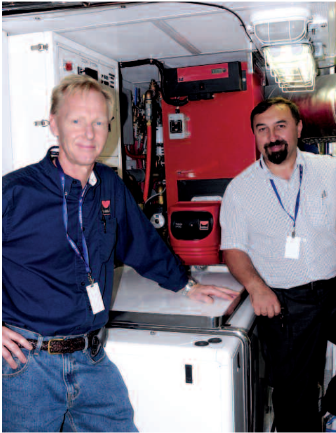
Above: MarineTec partners Lars Nilsson, left, and Costica Gheorghiu flanking a Kabola furnace. Right: A complete Kabola system installed in a lazarette aboard a new trawler.
