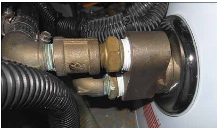
Water heaters equipped with heat exchangers can transfer waste heat from the engine to the water heater via the coolant. If installed near the engine, these units may deliver dangerously hot domestic water.
