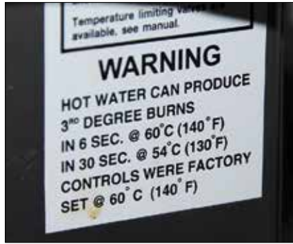
Above —Hot domestic water can cause serious burns, particularly if thermostats are set incorrectly, or if water is heated by engine coolant. In the latter case, mixing valves and anti-scald faucets can prevent dangerously hot water at the tap. Right —This infrared pyrometer is measuring the temperature of coolant as it enters a water heater.
