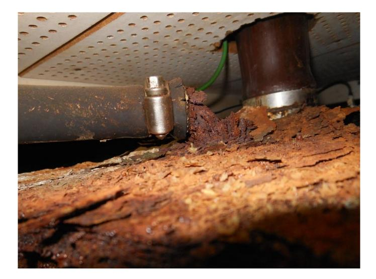
One of the more common forms of failure for steel tanks is from the outside in, or top down, the result of water leaks from the deck. Access to tanks, metallic tanks in particular, for inspection is, therefore, essential.
