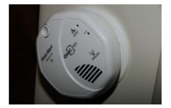
Linked fire alarms all sound if any of the alarms aboard detect smoke (and CO in some cases). These are especially useful when installed in locations where alarms may not be heard, such as engine rooms, thruster compartments and lazarettes.
