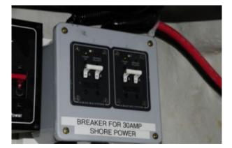
This professionally-installed AC-shore power circuit protection, installed within ten feet of the inlet, meets ABYC Standards. It is clearly labeled, installed in an approved enclosure, and indicates reverse polarity if the fault exists.
