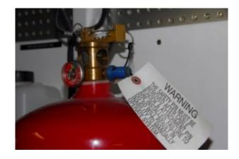
In spite of the large warning placard alerting installers to remove it, this fixed fire suppression system's shipping pin remains in place years
