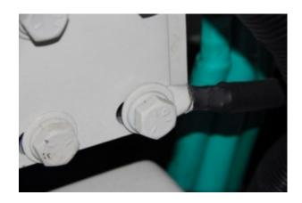
Installing electrical terminals over paint results in a poor, high resistance connection. This is a common occurance where ground and bonding connections are concerned.
