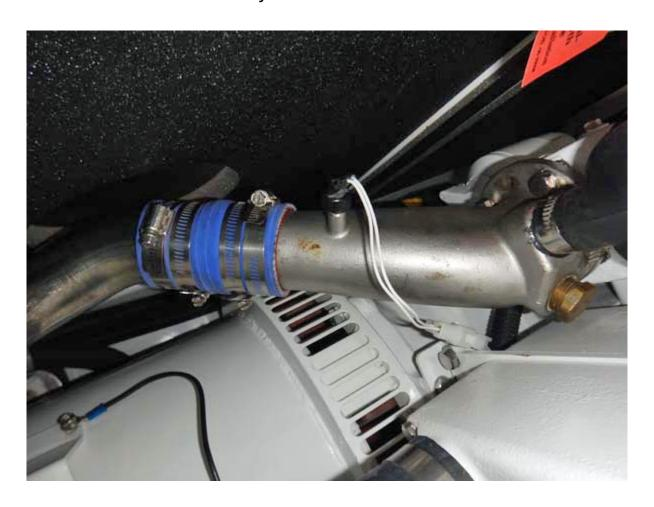
Most gensets incorporate automatic shutdown protection in the event of coolant and exhaust overheating, as well as low oil pressure. If any of these fail to operate while the genset is running the results could be costly and dangerous, particularly in the case of a failed high wet exhaust temperature shut down switch.
