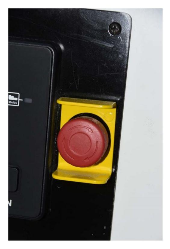
All gensets should have local start and stop, however, those equipped with an auto-start system must also have a lock-out feature, that when actuated will prevent the genset from starting until actively reset or released.
