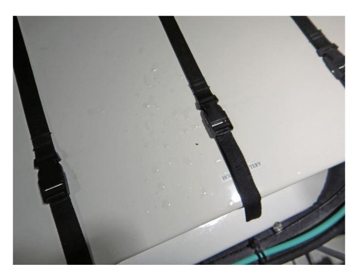
Light-weight straps and buckles have no place securing large battery banks.
