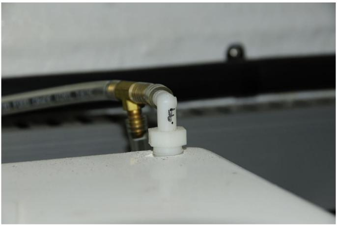
This battery box has been equipped with a remote ventilation
