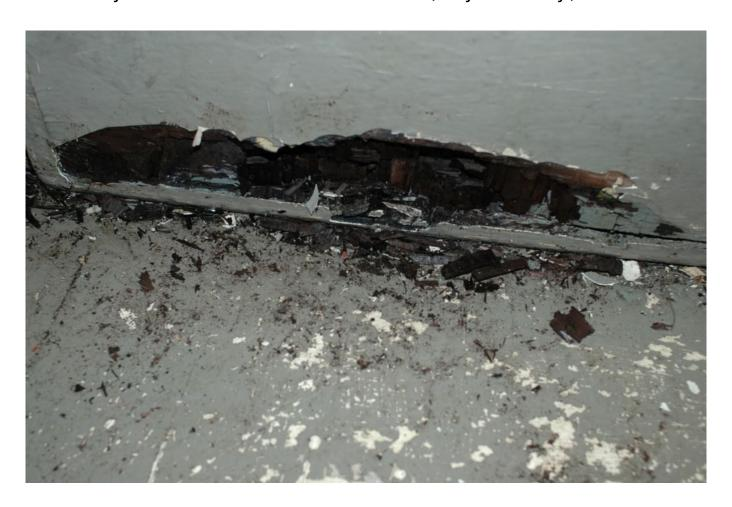
Raw or painted timber is unsuitable for battery box material, it is quickly destroyed by leaking electrolyte.
