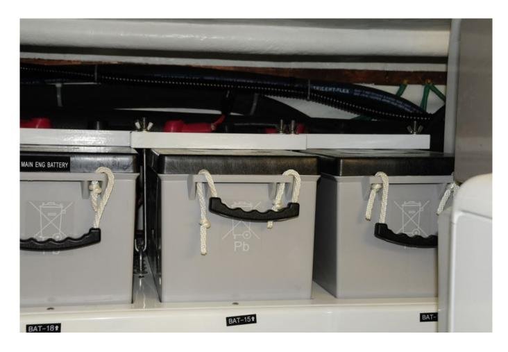
Clamped-down batteries, and through-bolted supports, with generous ventilation gaps, an installation worthy of praise.
