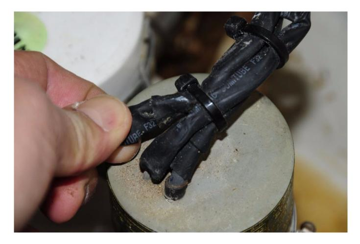
For unknown reasons, this float switch's connections were spliced adjacent to the switch. An attempt has been made to waterproof them, however, it's not one I'd trust, the switch should be replaced.
