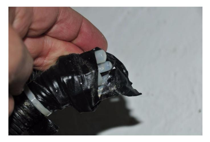
"Waterproof" means fully submersible. Connections like these, wrapped in electrical tape, will quickly succumb to immersion.
