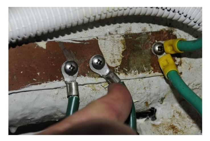
Tapping screws and thin copper strips are a poor combination, as they nearly always lead to loose, high resistance connections.
