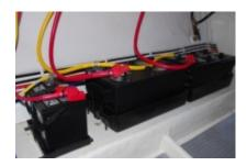
Starting and house batteries may require different methods for reliable load testing.
