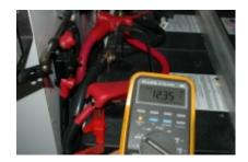
Although it will not test a battery's ability to deliver amperes, a high quality multimeter, such as the one shown here, will enable you to determine a battery's state of charge provided it's been, "rested". Based onthe voltage of 12.35,
