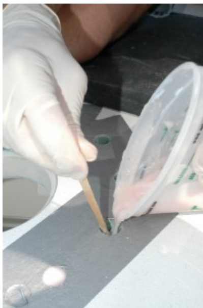
Filling the holes with thickened epoxy.
