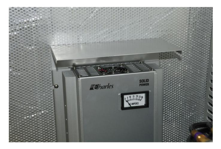
This battery charger manufacturer includes a drip shield as a standard component.
