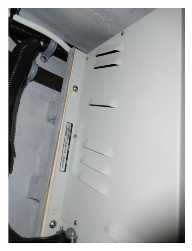
Louvers like the ones shown here can shed water, however, the cord grip beneath these is not water resistant.
