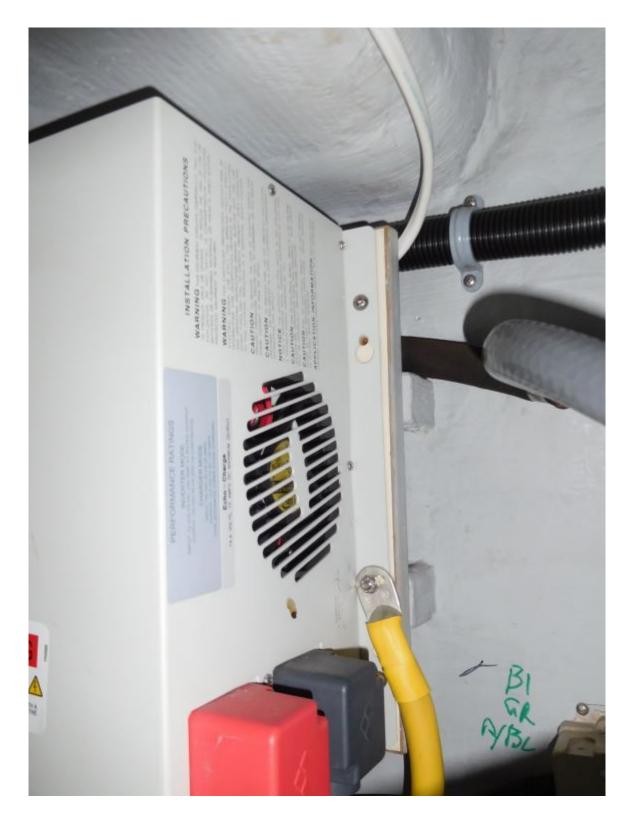
This inverter lacks a drip shield, its top and sides are louvered and thus open to water, and debris entry.
