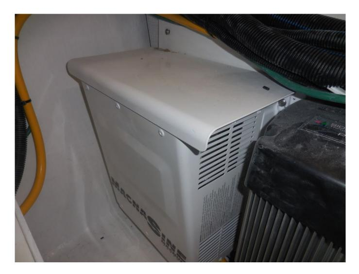
This inverter is equipped with an optional metallic drip shield supplied by the manufacturer. Note how it overhangs all of the sides.
