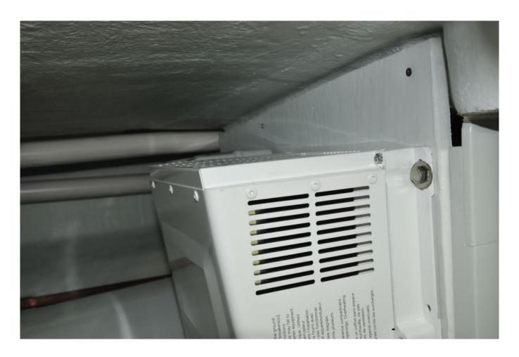
While these inverter installations look professional, the enclosures are louvered on their top sides; both should be equipped with a drip shield.
