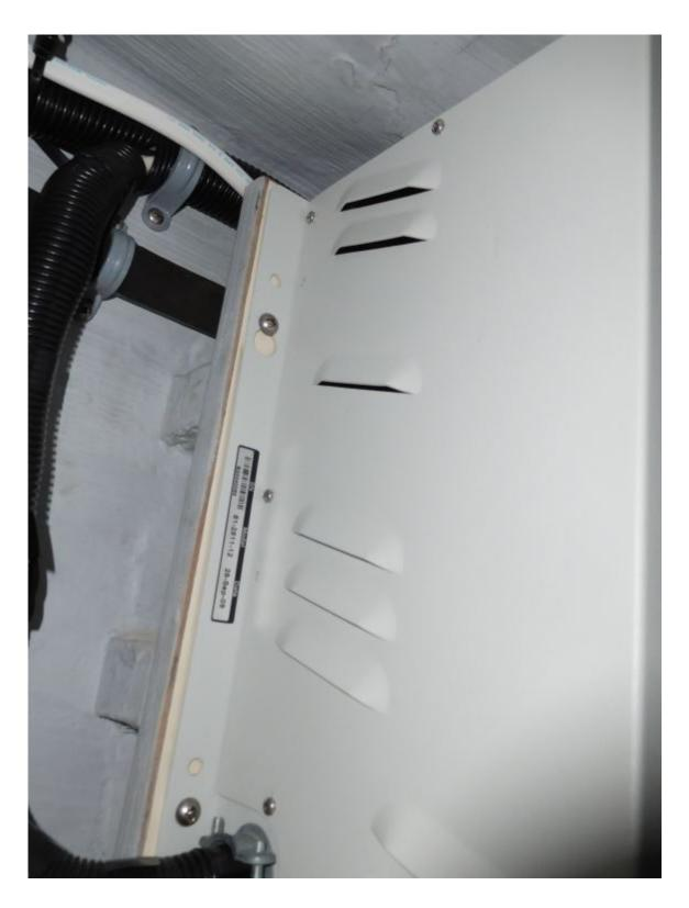
Louvers like the ones shown here can shed water, however, the cord grip beneath these is not water resistant.
