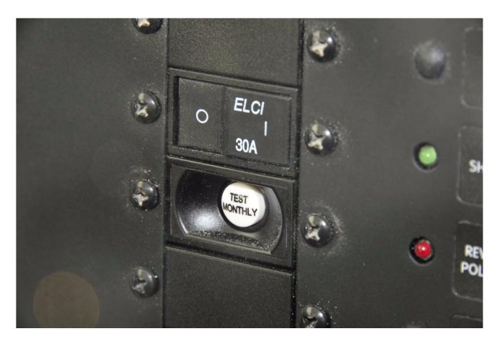
If the wire-run distance between the shore inlet and the circuit breaker panel is less than 10 feet, the ELCI may be located in the latter.
