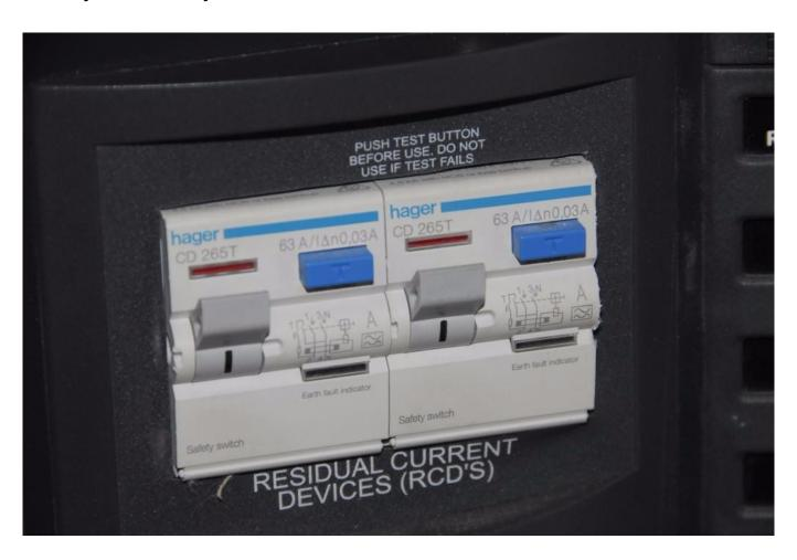
Like GFI's, ELCI's (sometimes referred to as RCDs) must include a test feature, the blue button with embossed T.
