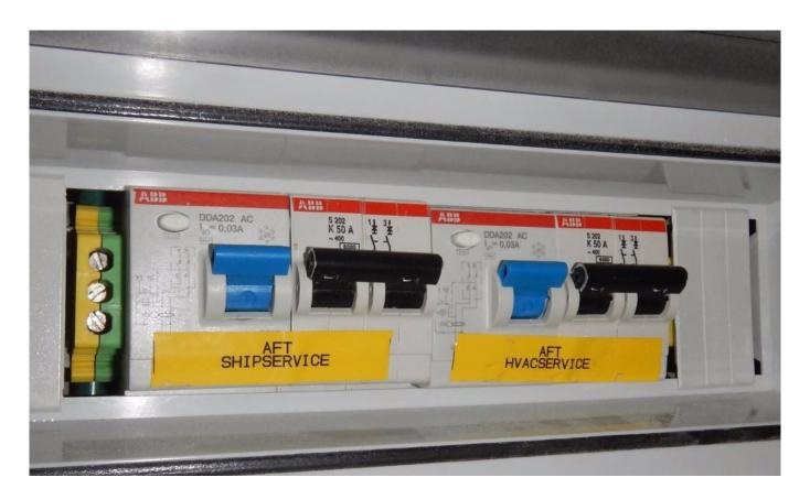
ELCI's, the blue-handles, are often combined or co-located with primary shore power inlet circuit breakers, the black two pole devices to the right of the ELCI. Don't assume an ELCI trip current is correct, as they are available in a wide
