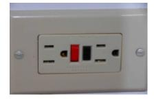
The humble and inexpensive yet ubiquitous GFCI receptacle is a veritable necessity aboard every boat. It's responsible for preventing untold injuries and saving countless lives both ashore and afloat.
