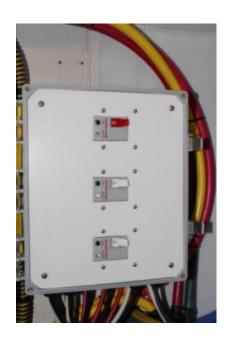
The RCD at he upper left is providing whole boat ground fault protection for this 30 amp, 120 volt shore power service. The Series of RCDs on the lower right are designed to afford ground fault protection for this vessel's 50 amp, 240 volt shore power service as well as the generator and inverter. Thorough protection indeed.
