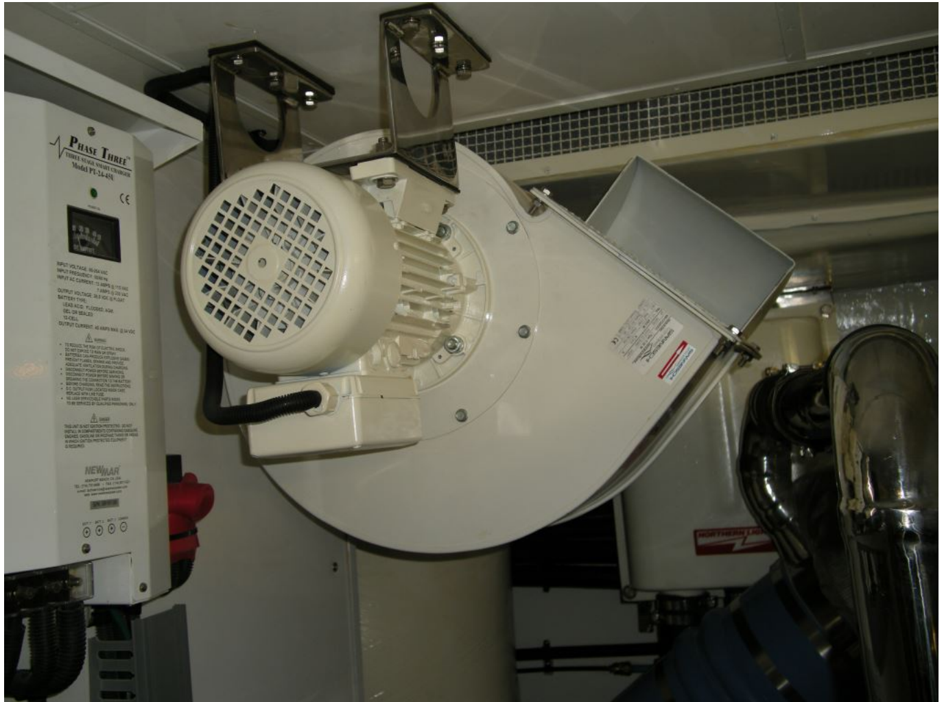
An industrial-size 'squirrel cage' blower. Units like these are designed to operate continuously, while at rest or underway.
