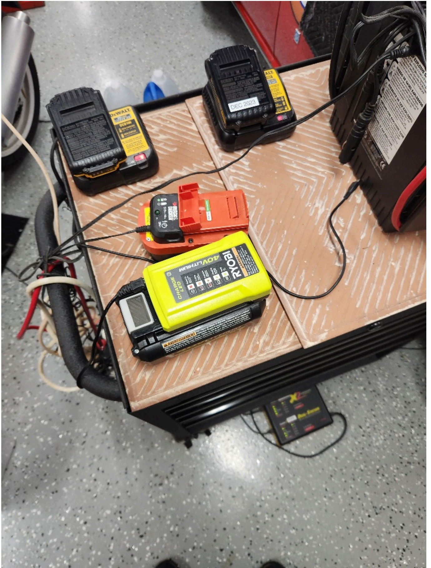
A ceramic top lithium ion battery charging station.
