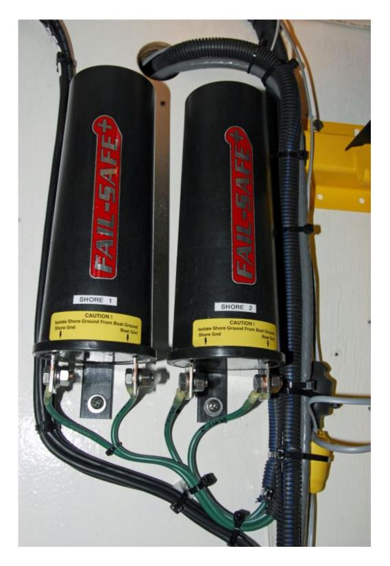
Galvanic isolators provide protection from galvanic corrosion that originates on other vessels, and comes aboard via the shore power cord's green grounding wire. They will do nothing to prevent stray current corrosion.
