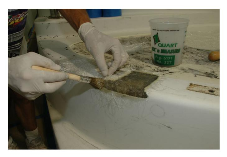
In order for a secondary bond to be reliable, the surface over which the resin and fabric are applied must be properly prepared.
