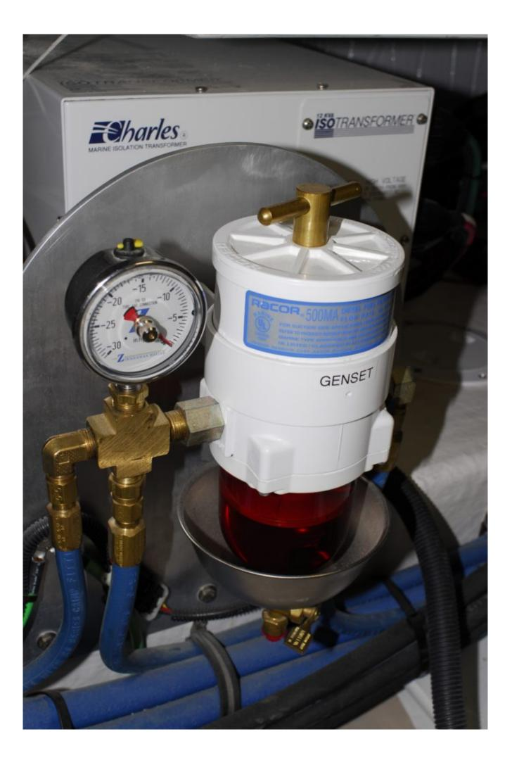
Primary fuel filter vacuum gauges provide the only accurate means of measuring fuel flow restriction. The arrangement shown here, with the gauge permanently plumbed to the outlet plumbing, represents the preferred approach.
