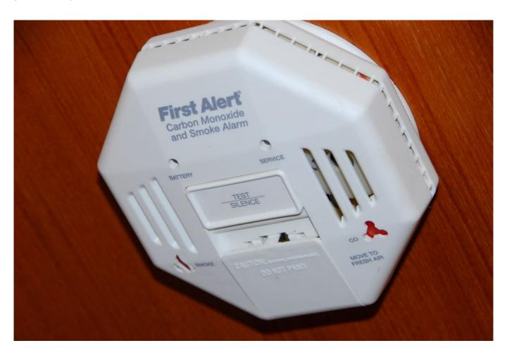
Fire detection; smoke detectors are cheap insurance, you should have one on both sides of every door aboard.
