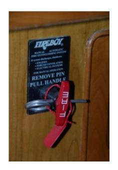
Manual discharge handles should easy to access, and located in plain view rather than in a locker or cabinet. If they are installed in a locker, a placard should be applied to the locker door indicating their presence within.
