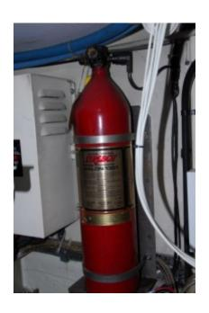
Fixed fire suppression system installation instructions should be followed to the letter, among other things, bottles should be securely mounted using through bolts rather than tapping screws, as well as being located high, on or close to the centerline and away from ventilation sources.
