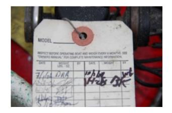
Systems should be periodically inspected by a professional. However, marine systems differ from typical portable fire extinguishers and not all inspection outfits understand or are able to scrutinize marine installations. Just because the inspection tag is initialed it does not mean the system has been properly inspected.
