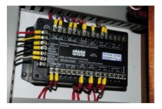
Automatic engine, generator and ventilation system shut down relay systems add complexity to a fixed fire suppression system, however, they are well worth the added effort.In order to remain ABYC compliant, this option is a necessity on diesel-powered vessels.
