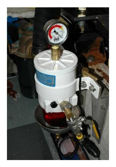
Ideally, fuel filter vacuum gauges should be installed in the outlet plumbing of single filters (top), rather than in place of the T handle (above). T handle gauge kits run several risks, including gauge damage and inaccuracy, and they make filter replacement more challenging.
