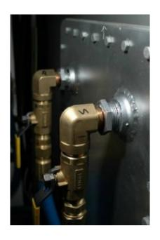
If polishing system supply and return fittings are located close together, a common installation fault, fuel will "short cycle", moving primarily between these two fittings, rather than across the bottom of the tank.
