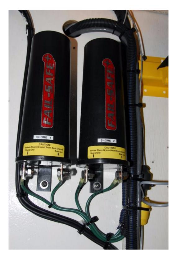
Galvanic isolators present an effective means of limiting DC current flow over shore power ground wires, thereby diminishing the likelihood of galvanic corrosion occurring as a result of interaction with nearby vessels or metallic dock structures.
