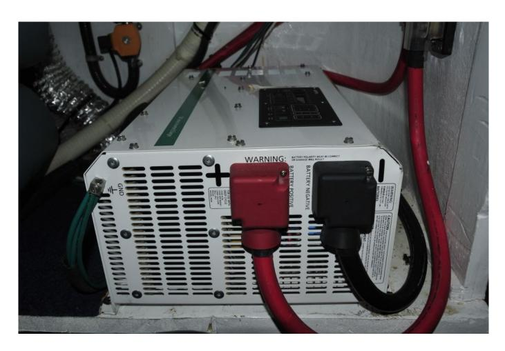
Most inverter manufacturers clearly establish the proper mounting orientation in their installation manuals. Inverters should not be installed with vented or louvered surfaces facing downward. This inverter is installed incorrectly; the downward facing panel is vented, which would allow hot or burning material to fall through the case, onto the wood shelf beneath, in the event of an internal fire.
