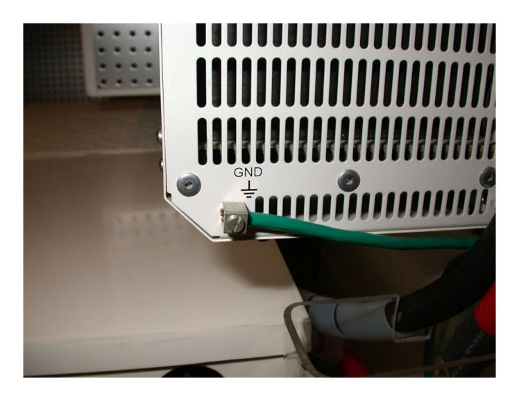
Under-sized chassis grounds are among the most common installation faults. Not only us this chassis ground wire undersized, its lug is also of the direct bearing variety, i.e. the screw turns directly against the wire's strands, a clear violation of ABYC standards.
