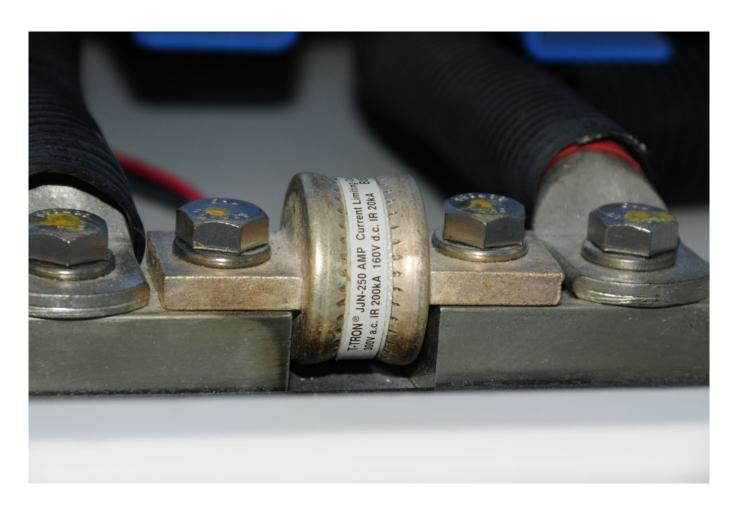
Nearly all inverter manufacturers call for the use of specialized "Class T" fuses. Failure to use the correct fuse can lead to nuisance tripping or, worse, failure to interrupt current flow in the event of a short circuit.
