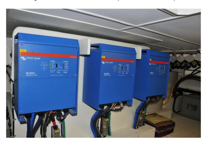
"Stacked" inverters, which are growing in popularity, afford users the ability to operate a vessels electrical system in a near-seamless manner with shore power and generators.
