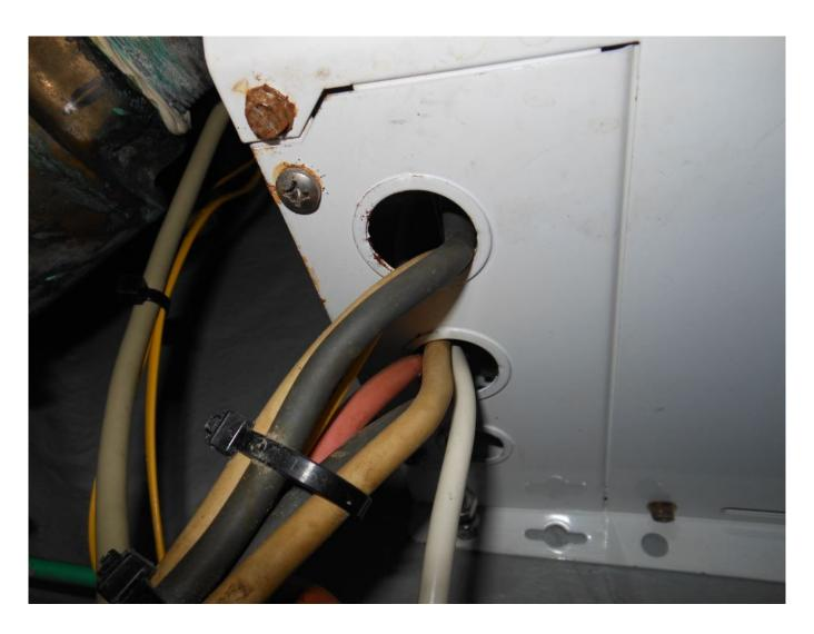
Yet another all too common installation fault, failure to use proprietary strain relief connectors, or "cord grips", the result of which is a serious potential for a short circuit or electrocution.
