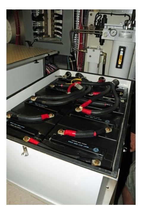
The size of capacity of a house battery bank should be inextricably linked with the expected inverter loads. Failing to take this into account will often lead to frequent charging and shortened battery life.
