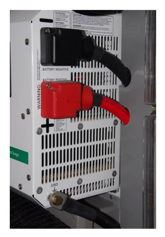
A dramatically undersized chassis ground, top, and a properlysized chassis ground, above. Failure to utilize the correct gauge cable for this application could lead to overheated wiring and fire.
