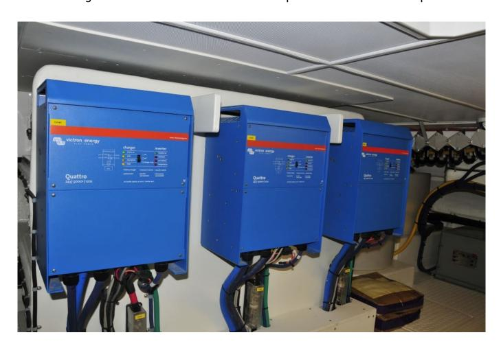
"Stacked" inverters, which are growing in popularity, afford users the ability to operate a vessels electrical system in a near-seamless manner with shore power and generators. This installation lacks ABYC compliance in that no drip shield has been installed (the IP rating on these inverters is 20, more on that here). Unless the inverter has inherent drip
