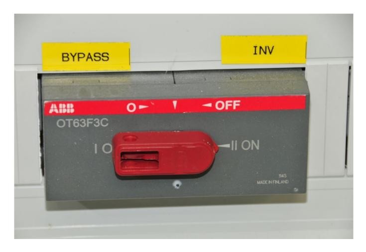
While inverter pass through relays are typically very reliable, a failure could prevent shore or generator power from flowing through an inverter, supplying the inverter bus loads. For that reason, some builders opt for an external bypass switch.
