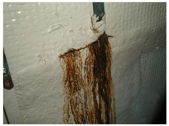
When brown "coffee staining" like this shows up, it's obvious that water has penetrated the core. In this case a moisture meter would be used to identify the extent to which it's spread.
