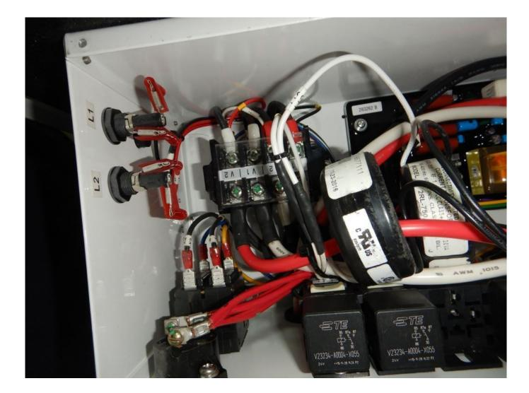
Generators and inverters are a source of power, and thus when they are producing power, their neutral and ground wires must be bonded to each other.
