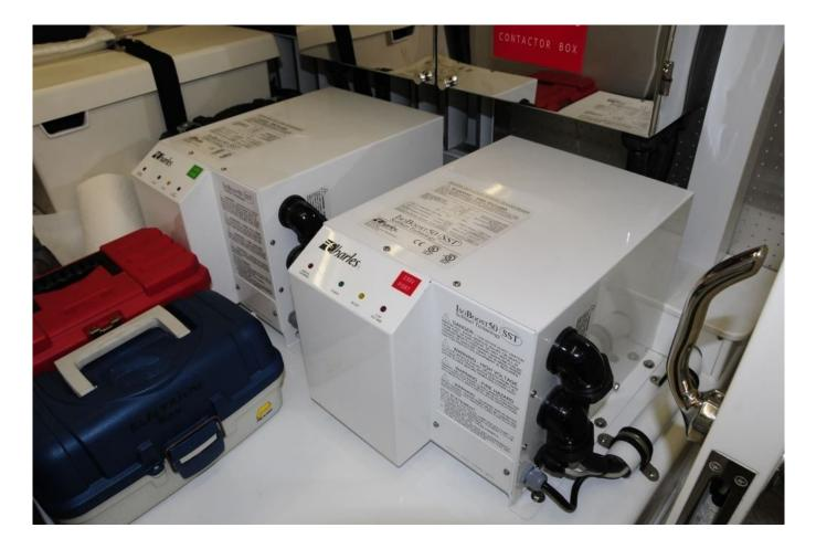
Shore power transformers provide an added measure of safety, and virtually eliminate the safety issue associated with neutral to ground connections.
