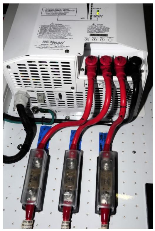
A common over-current protection error, installing the fuse adjacent to the consumer or appliance rather than the power source.
