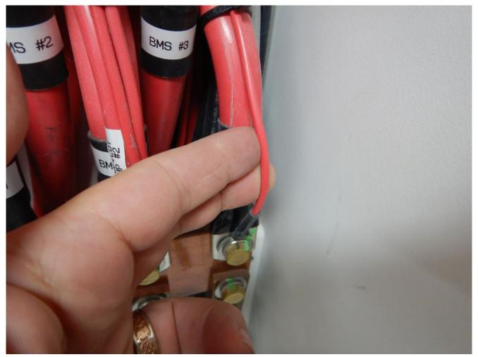
It's not necessary to know what this wire supplies power for to know it's in violation of the OCP standard, it's connected to a distribution bus, and it lacks over-current protection within 7-inches (metallic rings should be removed when carrying out electrical inspections or work).
