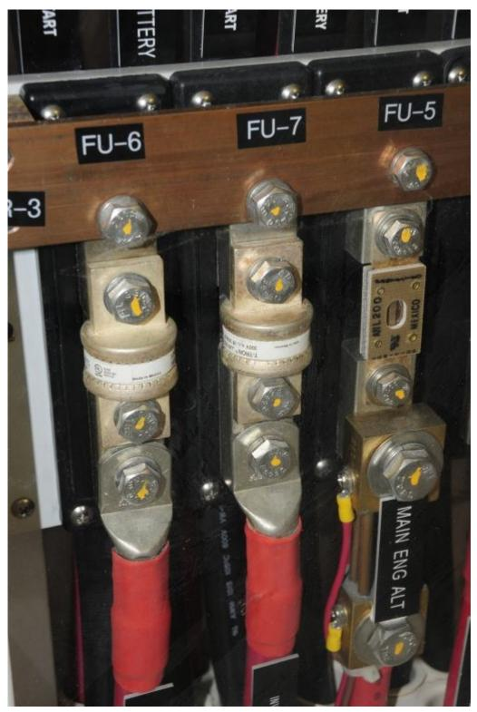
Fuses and circuit breakers should be placed as close to the source of power as possible, this includes batteries and other distribution points like the bus bar shown here.
