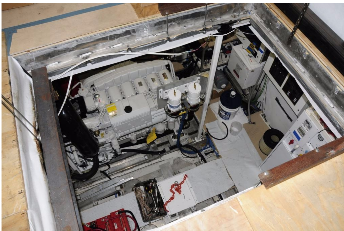
The nearly completed engine room, viewed through the soft
