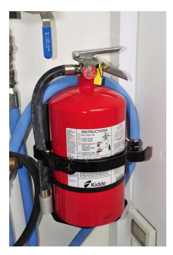
Portable fire extinguishers should be chosen based on the type of fire they may be called upon to fight, as well as the location. It makes sense to place large capacity extinguishers, like the one shown here, in engineering spaces.
