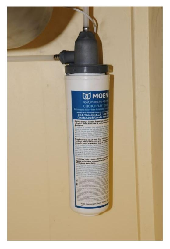
Point of use filters offer an added measure of water cleanliness, for drinking and cooking. Most are installed under counter tops, with a dedicated spigot.
