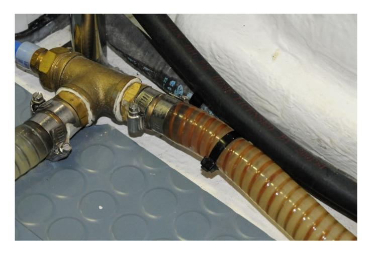
Clear hose is less than ideal as it will support algal growth. This hose is also not rated for pressure applications, it's bulging between its wire reinforcement.
