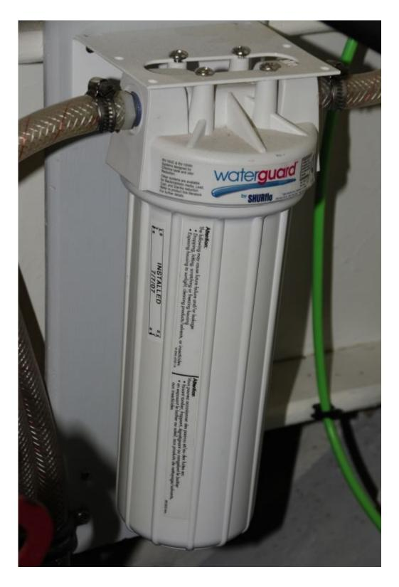
Whole-vessel filters provide filtration for all water leaving the vessel's tanks. Canisters, and replacement elements, of this sort are readily available, and inexpensive, t home improvement stores. They should always be installed after pumps.
