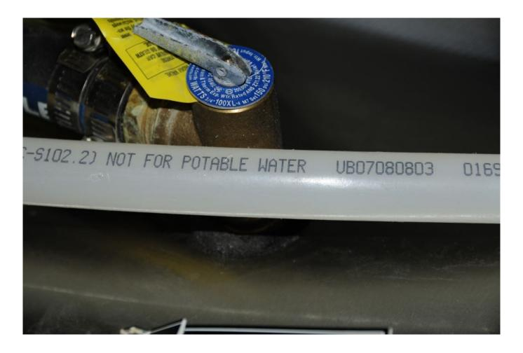
While some hose may appear to be appropriate for potable water use, check carefully and don't assume that a hose is suitable unless it's been identified.
