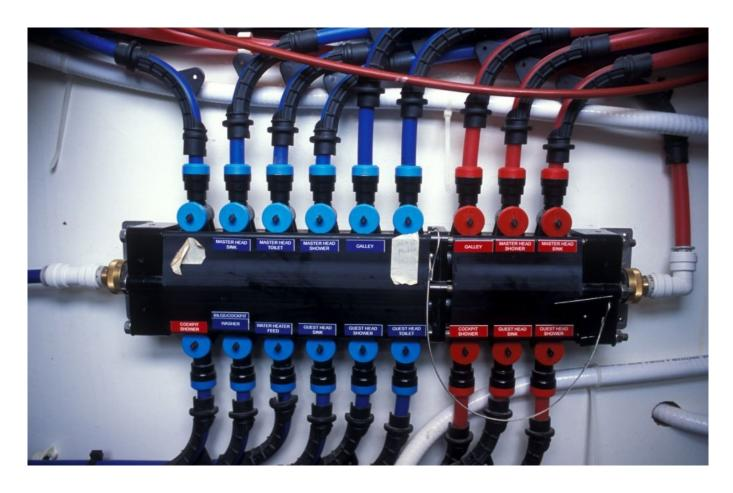
Proprietary polyethylene plumbing systems like the one shown here have become increasingly popular, they are leak-
