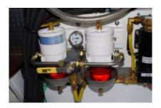
Tandem filter arrangements offer the user the option of keeping a clean filter in ready reserve at all times.
