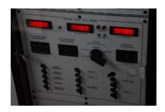
Monitor your AC panel ampere meter to ensure proper break-in load.
