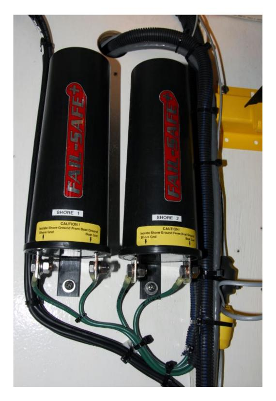
Every vessel that is equipped with shore power should utilize, at the very least, a galvanic isolator, like those shown here, if not an isolation transformer. If your bonding system is not isolated from the dock ground, your anodes could end up protecting vessels that are adjacent to yours.
