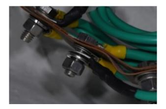
Ideally, this bonding "bus" should utilize a purpose made bus bar rather than copper strap material. The loose center log represents potential high resistance, which could prevent this component from functioning properly and safely.
