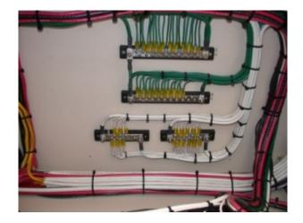
There is no connection between the green grounding and white or neutral AC wiring at these bus bars. Care must be taken at installation and through all future service that, except for a few isolated cases, the two circuits remain separate aboard the vessel.
