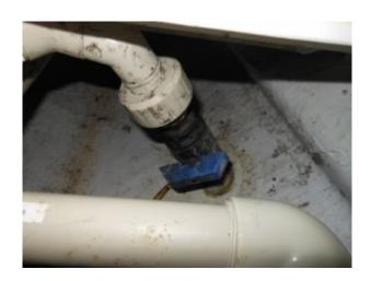
This "seacock" is in fact a polyethylene irrigation valve, making it inappropriate for use as a sea valve. The rigidly attached PVC plumbing imparts leverage to the installation, further jepordizing its reliability.
