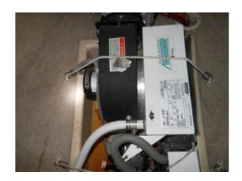
This self-contained air conditioning unit weighs 56 pounds and is installed relying solely on 1/4" bungee cord. One can
