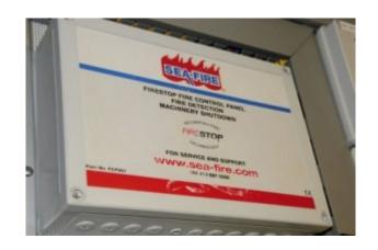
Central station smoke and heat alarms (this one also shuts down engines, generators and ventilation systems in the event the engine room fixed fire extinguisher is discharged) are valuable indeed, and ideally suited to new builds.
