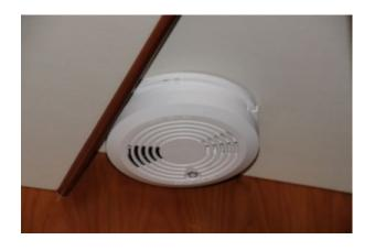
A closed door can negate the effectiveness of a smoke alarm. Thus, for the cost, smoke alarms should be placed throughout your vessel, including on both sides of every door.
