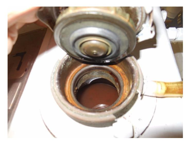
Because they must maintain an air void within when not used with a recovery bottle, steel and cast iron expansion tanks are prone to rusting.
