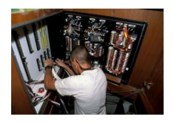
Electrical systems in particular have grown in size and complexity, placing a greater emphasis for compliance with vessel manufacturer and ABYC Standards when carrying out repairs and modifications.
