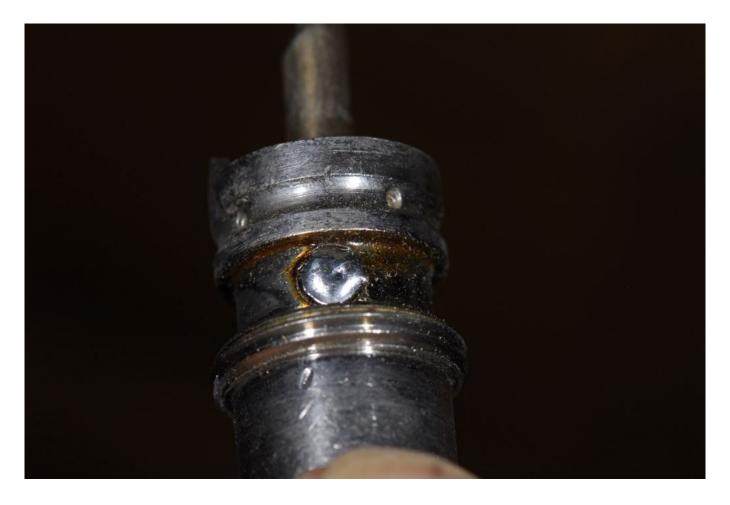
Proper solder joints, like the one shown here, are critically important. These can be difficult to achieve if inadequate heat is available when, for instance, the termination is being made outdoors, in breezy conditions.
