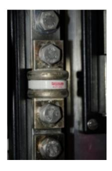
Over current protection, fuses and circuit breakers, must be installed as close to the battery as possible, within 7 inches for American Boat and Yacht Council Standards compliance.
