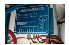
External, multi-stage, temperature compensated "smart" regulators make all the difference when it comes to controlling high output alternator. The internal regulator supplied with most stock alternators has a reliable but unsophisticated charge profile or voltage range. In spite of the alternator's rated output, when guided by such a regulator, it's simply not capable of replacing
