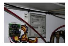
A single regulator controlling two alternators with the help of an intermediate controller.
